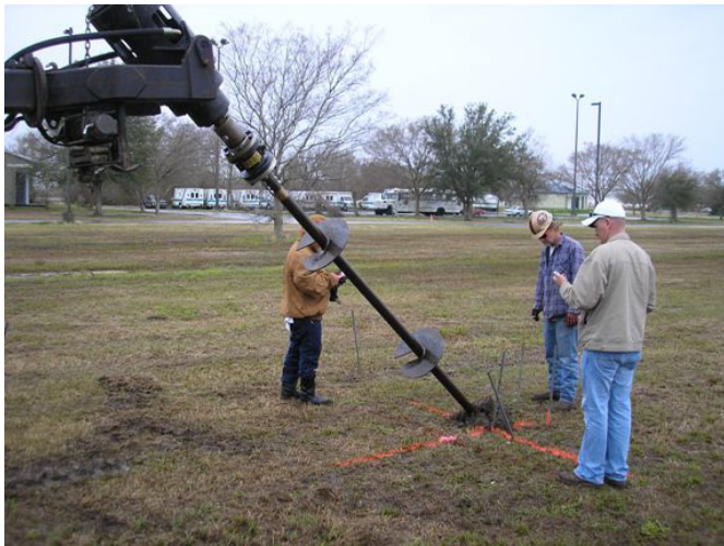
Figure 2: Installation of helical anchor (photo courtesy of Viking Helical Anchors).
